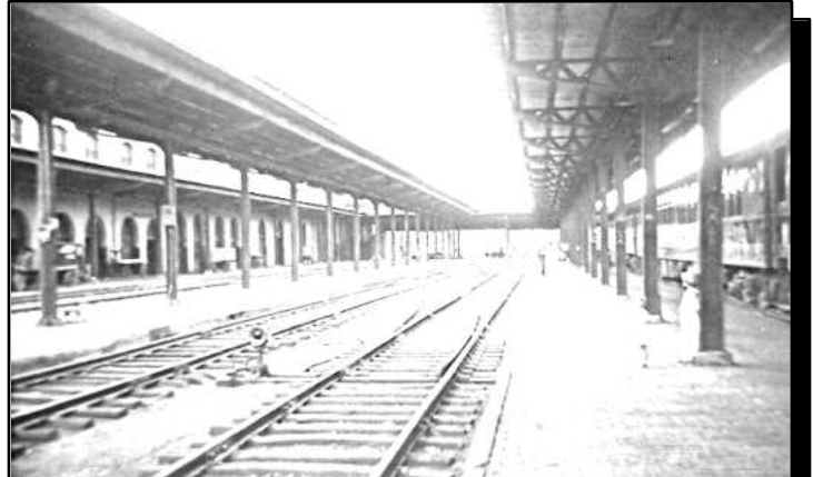
Duluth Union Depot (GN and NP) abounding with platform details and track layout. Nice touch with small boy and his sister waiting for a train.
