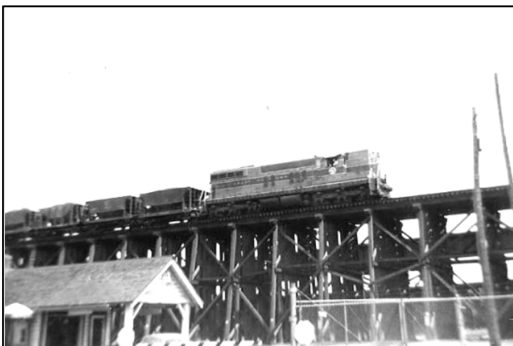
A GN SD-9 shoves a string of loaded ore cars onto the huge Allouez Docks in Superior, Wisconsin, in the summer of 1958.
